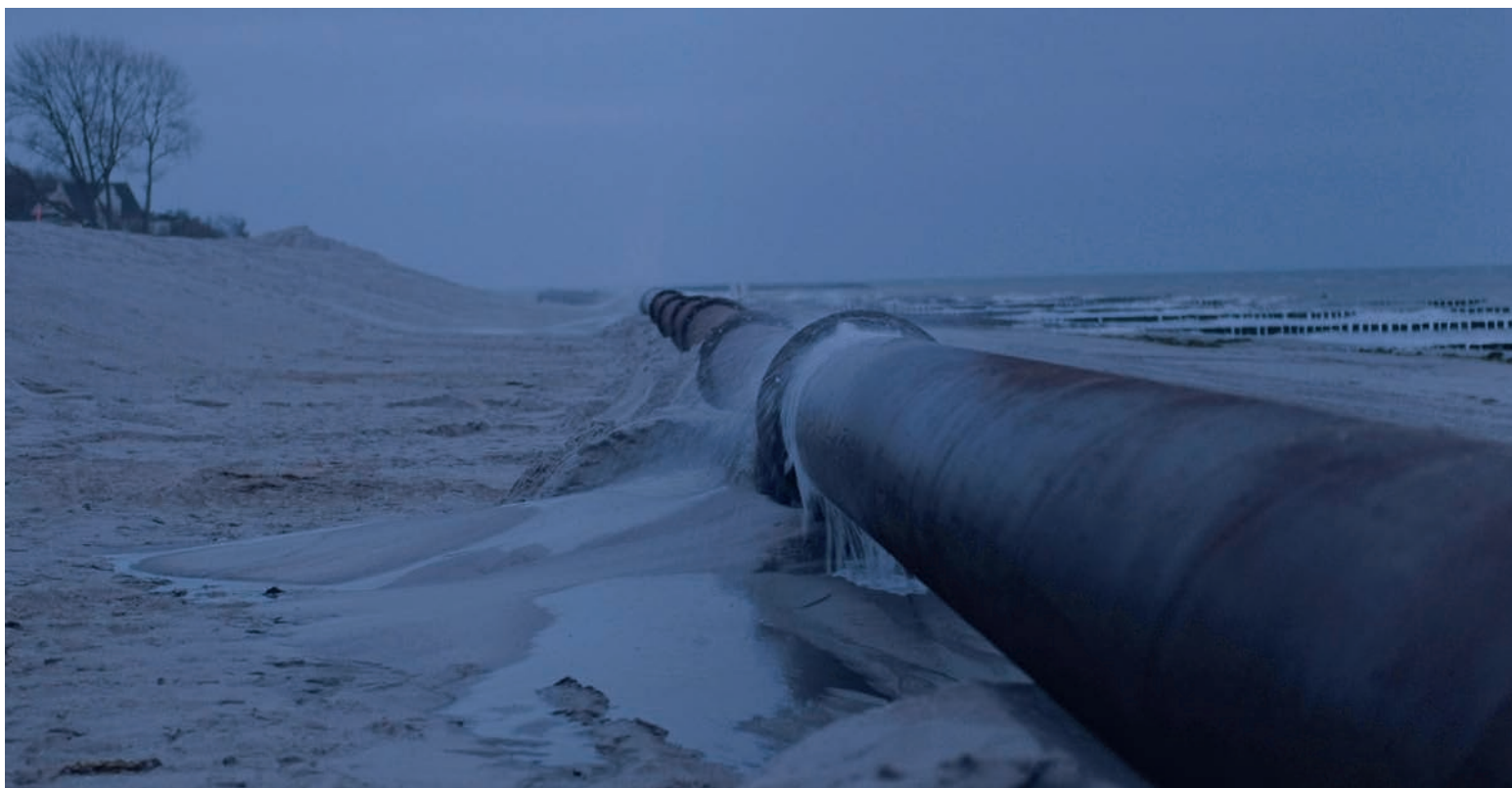
The sand is pumped through a pipe and distributed on the coast. Film still. Assembling the Coast. 2022.
